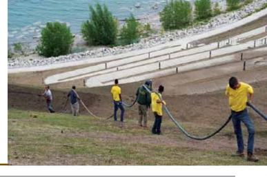
vertical drop distance (nearly 140 ft) the product slurry was applied through several sections of 3-in. hose and a specialized nozzle. A second application of Verdyol's Virgin bonded fiber matrix (BFM) was applied for enhanced erosion control, thermal and moisture containment, and vegetation growth enhancement. The BFM application reduced the watering frequency requirement, thus reducing costs.
